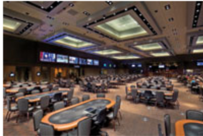
The videowall at Talking Stick Resort and Casino is comprised of six Panasonic TH-103PF9UK HD 103in. plasmas. Forty sources feed content to the screens regularly.
